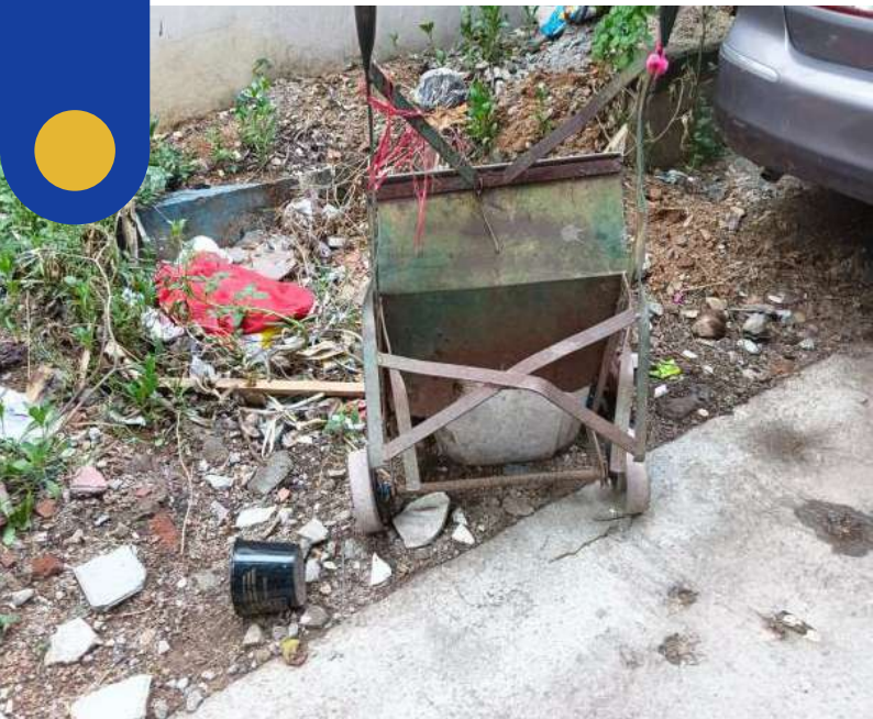
STATUS OF RWHS BEFORE RENOVATION
